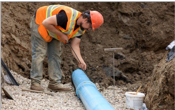
Figure 8. Insertion of Spline into Spline Lock PVC Pipe
