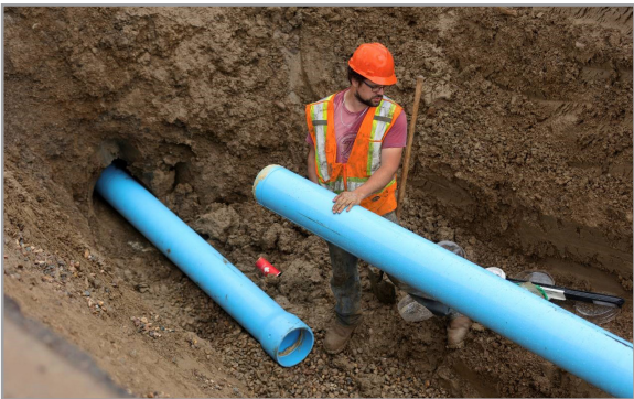
Figure 7. Assembly of Spline Lock PVC Pipe
