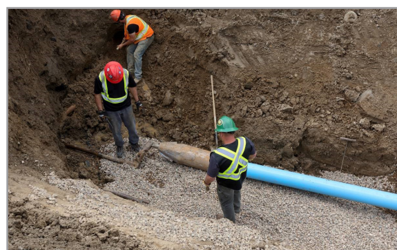
Figure 6. Attachment of Pipe Bursting Expander to Bursting Rods
