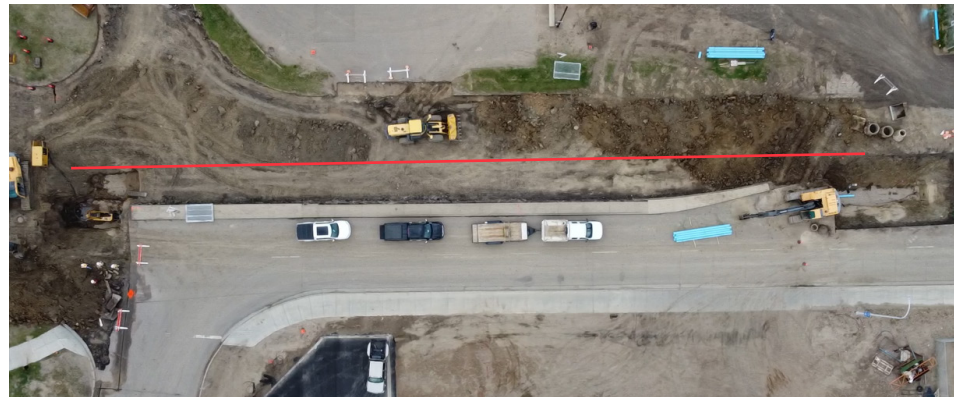
Figure 2. Aerial View of 200mm (8 in) Sanitary Pipe Bursting Installation – 62 nd Avenue
