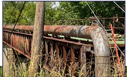
ORIGINAL STEEL WATER PIPELINE
