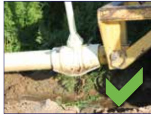
Connecting to tractor to break pipe free for removal
