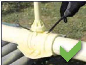
Insert pointed end of spline first
