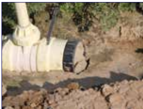
End plug to be removed
