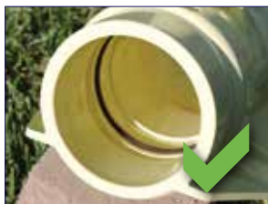
Properly installed O-ring
