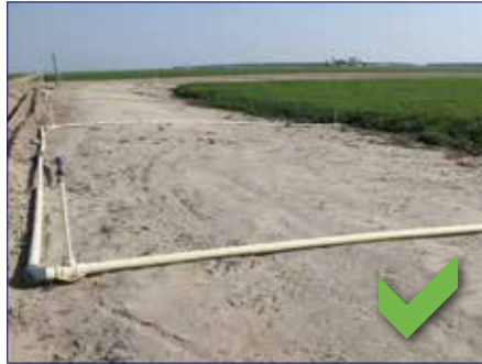
Certa-Set pipe entirely installed in a "U" design pattern
