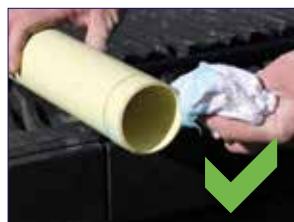
Applying lubricant
