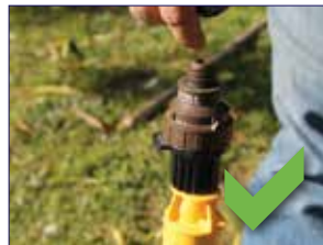
Place [MRDC] [MR] or [MDC] onto riser first
