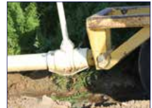
Final connection to tractor to remove/move pipe
