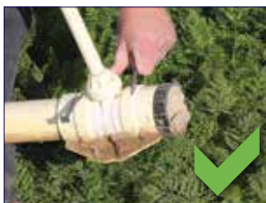
Remove spline
