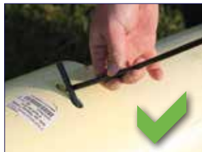
Push spline into the spline hole
