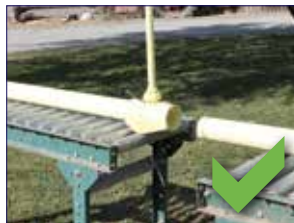
Pipe roller table setup
