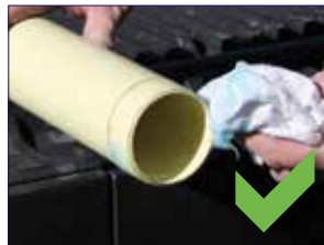
Applying lubricant
