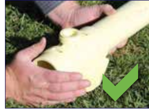
Push sled coupling onto pipe
