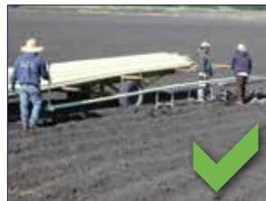
Pipe roller table setup
