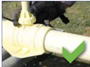
Insert pipe into sled coupling
