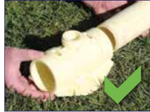
Push sled coupling onto pipe
