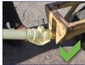
Connecting pipe to tractor
