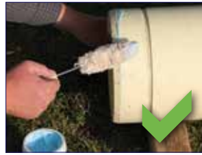
Lubricate spigot
