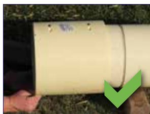
Properly aligned pipe and coupling
