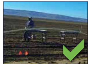
Pipe roller table setup
