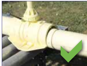
Insert pipe into sled coupling
