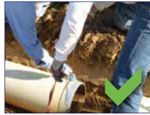
Lubricate spigot
