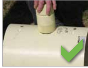
Tapped coupling assembly
