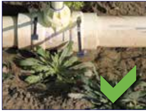
Silt and foliage surrounding sled coupling
