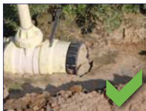
End plug to be removed
