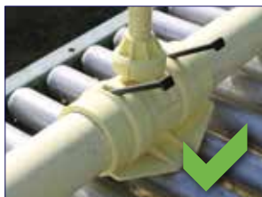
Correctly inserted splines
