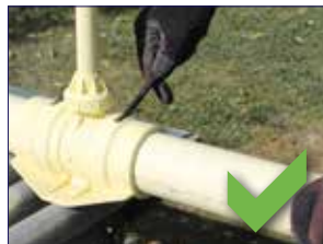
Push spline into the spline hole
