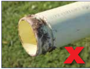
Pipe with debris
