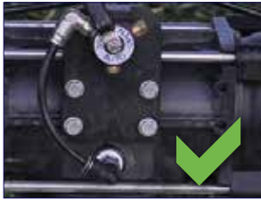
Nelson valve installed onto tapped coupling
