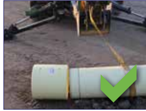
Backhoe with a strap
