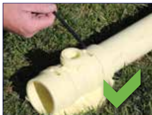
Insert pointed end of spline first
