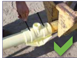
Connecting pipe to tractor
