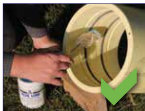
Applying lubricant
