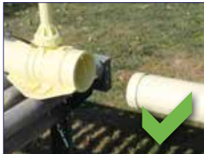
Insert pipe into sled coupling
