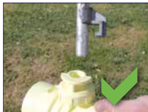
Align riser with riser cap
